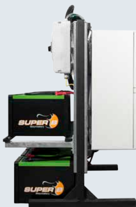
8Kw Off Grid system with Li-ion batteries
